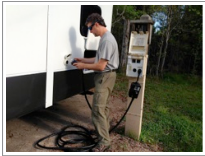
Mike connects the RV to Campground Power
